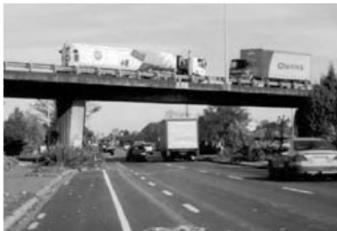
7. Southern Motorway Christchurch Grade Separation Lincoln Rd, opened 1977, M.Douglass
