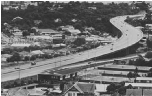
3. Newmarket Viaduct 1963 Auckland motorway - NRB
