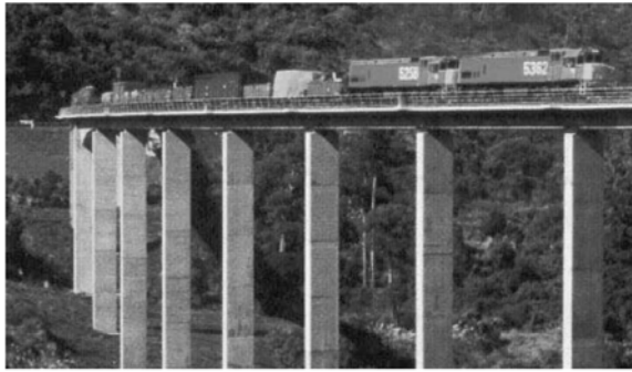
1. A Main Trunk Viaduct opened 1987 Near Taihape - Mark Cole
